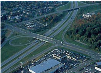
Aerial image at I-675 and SR 48 intersection looking southwest
